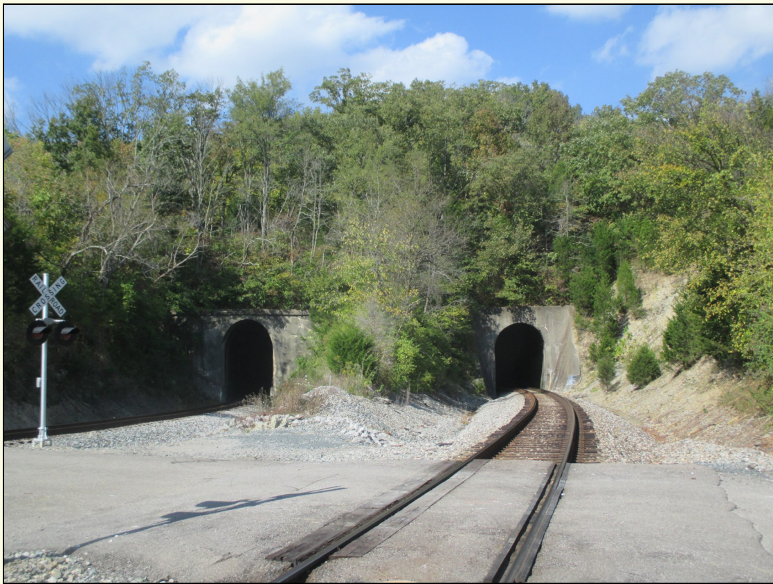
The Twin Tunnels at Grants Bend
